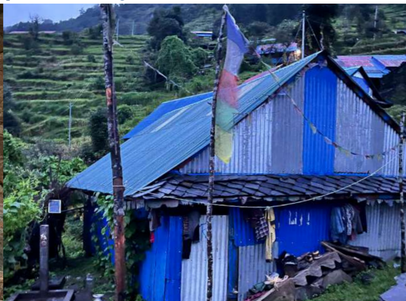
Figure 21 Typical house built with tin sheets, the traditional stone slates roofing tiles are occasionally used
